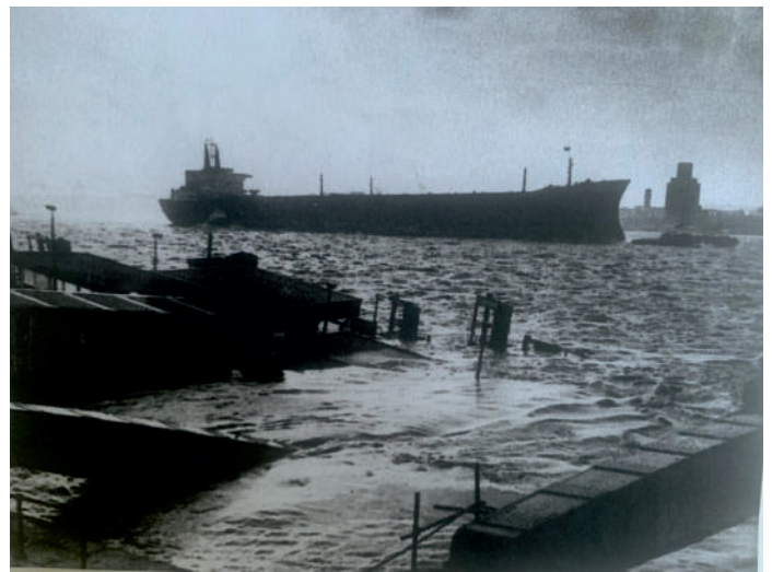
Above: the collapsed landing stage
