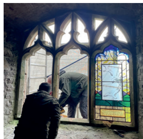
Below: Installation proceeding slowly!
